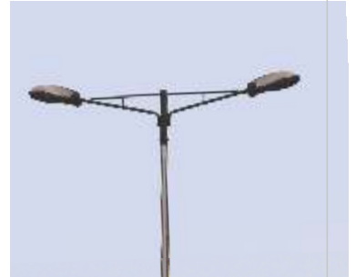
Western Express Highway, Mumbai
