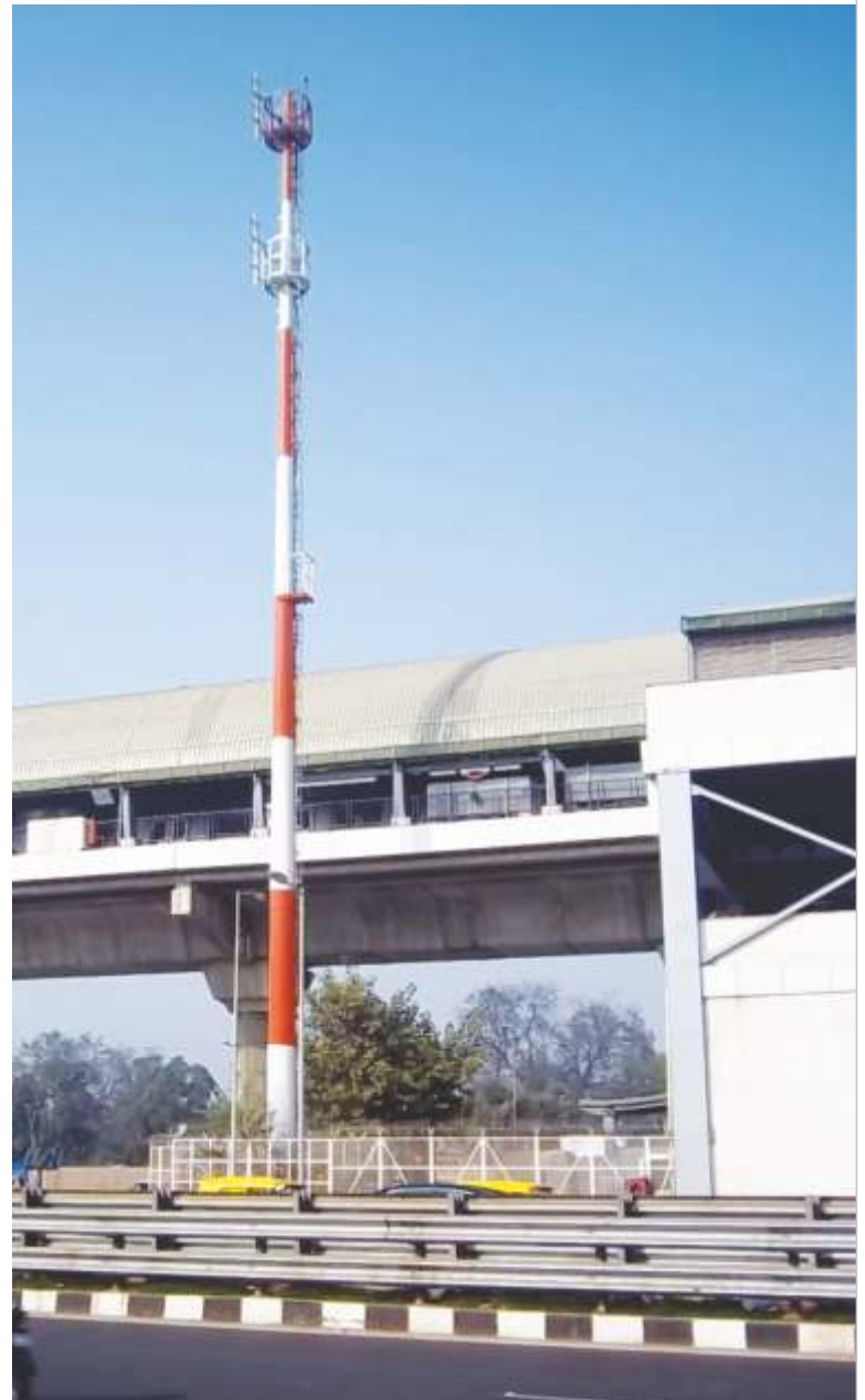
Design, Engineering, Supply, Installation and Commissioning of Radio Tower for DMRC, Delhi
