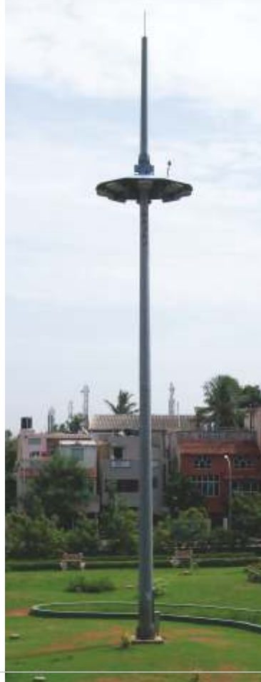
Design, Engineering, Manufacture and Supply of Umbrella Mast at Katipara Junction, Chennai
